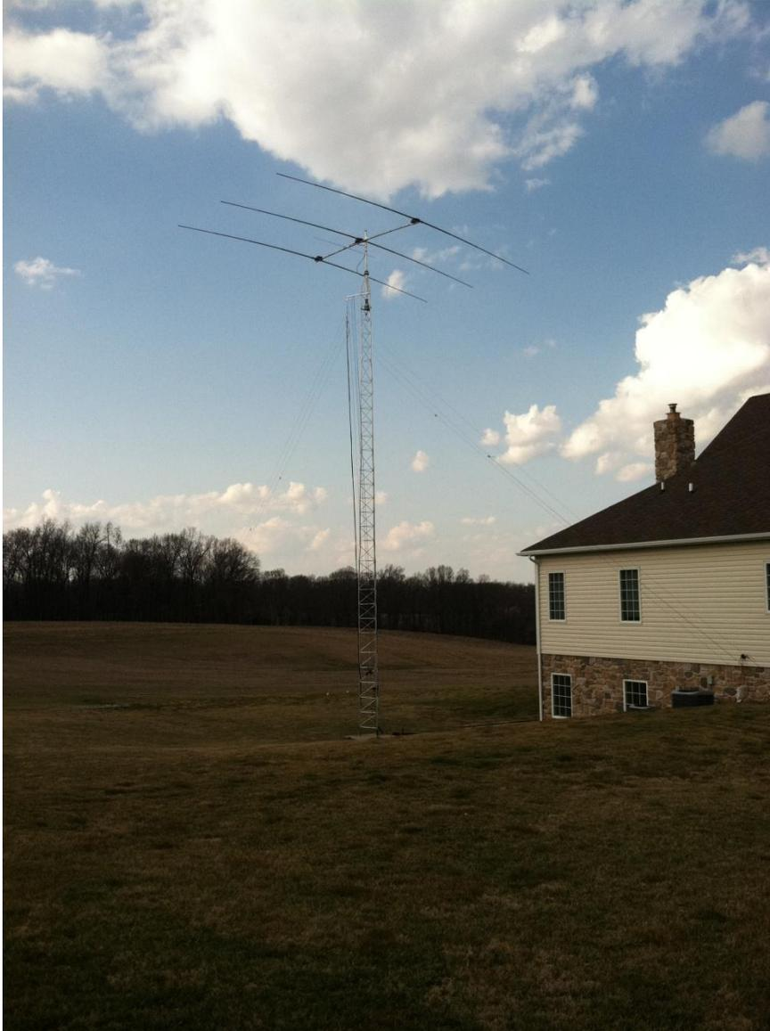
The finished product - 3-element SteppIR at 50 ft. along with inverted V's for 80,40 and 30."
