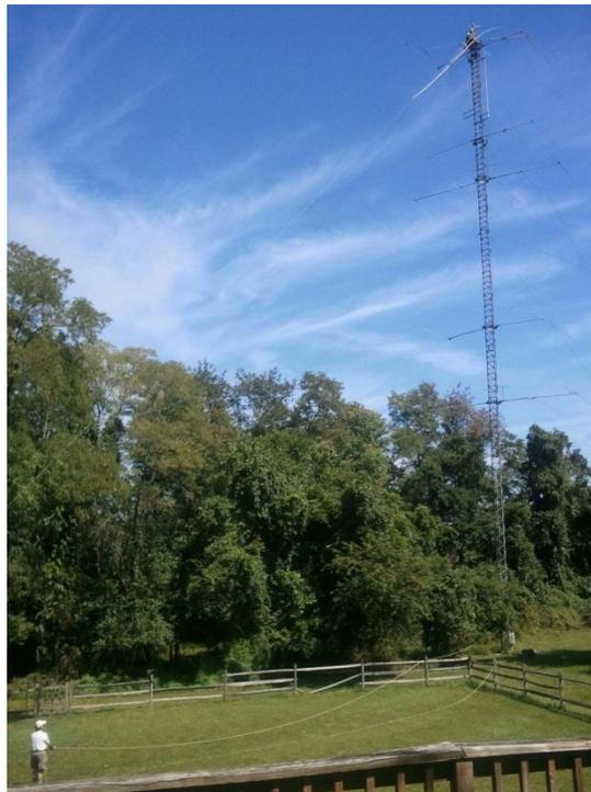
With Mike standing at the 134 foot level on the top of the tower, we rigged my stainless steel cable tram line, tensioned it to about 800 pounds. Mike attached the EF-180C to the tram pulley and we lowered it to the ground. While Mike waited on the tower, I replaced both element tips, riveted them in place, and hauled the antenna back to Mike using my lawn tractor to pull it back up the tram line. Mike reinstalled it on the mast, raised the mast, secured it all and I was back on 80m big time!
