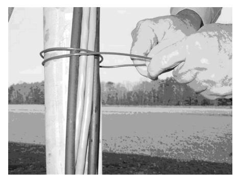
Here's step one: measuring, cutting, and then wrapping the wire around the tower leg. It's important that the backside of the wrap (the side away from you) not be crossed—it should be two separate, smooth wraps. You can draw the wires together in the front and cross them.
