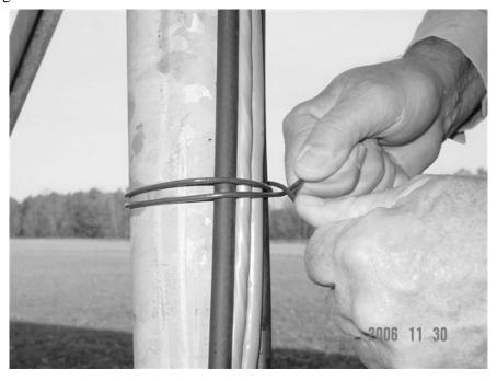
Pull the wires tight and begin to wrap the ends together.
