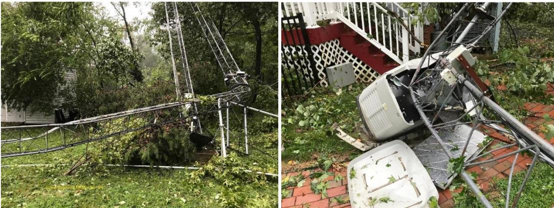
The whole house generator still started even after the tower smashed it. Unfortunately, it didn't provide any electricity. Had to go outside in the wind and rain to shut off the gas going to the generator to get it to stop. The good news is the commercial power came back on after being out for less than seven hours.
