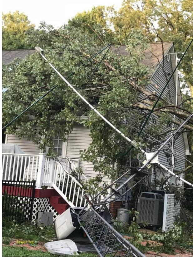
The "Tower Top" picture shows a tree on the house roof, wiped out generator, the tower top, the remains of a 4-element SteppIR, a 40m Moxon and the bent 2-inch dia., 1/4 inch wall, chromoly steel galvanized mast. The tree saved much more damage to the house by absorbing the falling top of the tower rather than the house.
