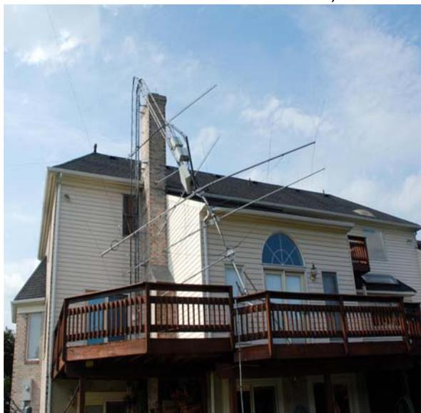
This picture shows what greeted us on our return from a trip to Russia on August 26 - apparently two days after high winds had hit parts of Clarksburg MD. The tower was 50 feet of Rohn 25G, of which the lower 30 feet were securely bracketed to the masonry chimney. It buckled just above the topmost bracket.
