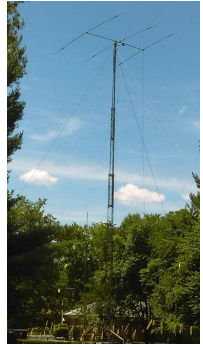
Portable crankup tower with TA33 and apex of 80M delta loop at 60'
